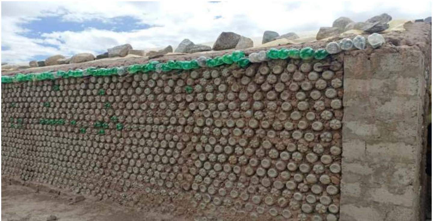
A greenhouse made from recycled plastic bottles, Kirti
